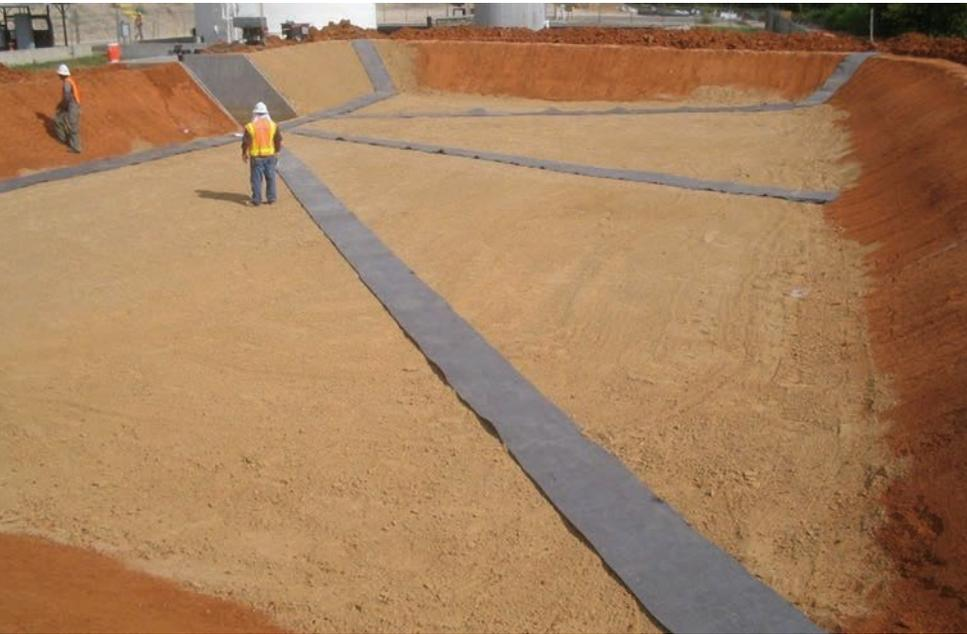
**Figure 3** Construction using gas-venting strips below a pond liner
